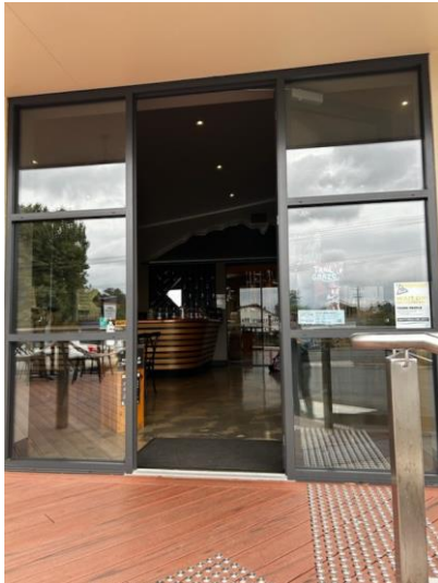
Main Entrance Door
