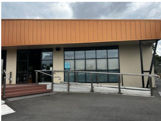
Main Entrance Ramp and Stairs
